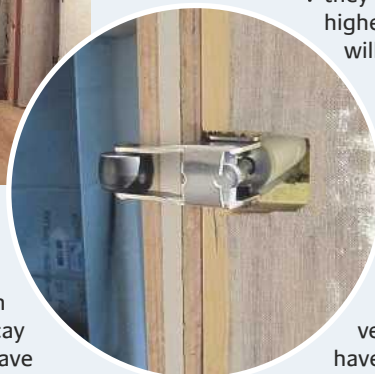
ABOVE: This latch ensures the door to the room closes with a perfect seal
