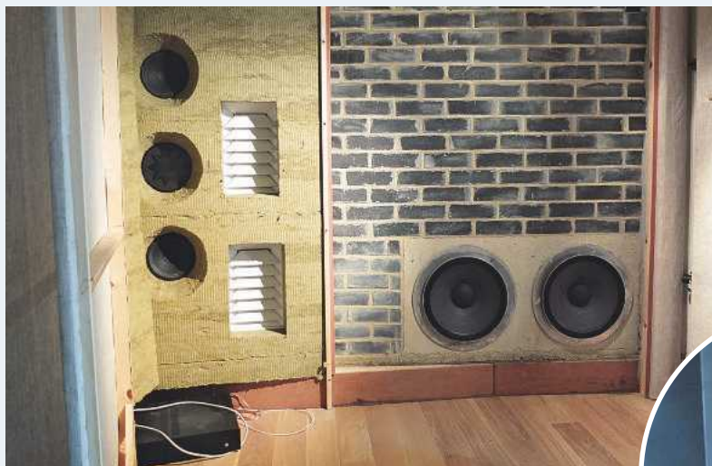
LEFT: In Michael's listening room, massively constructed subwoofer enclosures are positioned at crucial angles. There are no parallel surfaces
