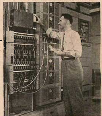
To keep colors true in television, signals must be kept on one of the world's strictest timetables. Equalizers that correct off-schedule waves are put into place at main repeater stations of the transcontinental radio-relay system.
