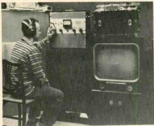
Fig. 5 (left). With hand on record-level control, operator is positioned to set proper level for recording while he monitors with earphones through phone jack. Fig. 6 (right). With both hands on editing knobs, tape is jockeyed slowly through head assembly to spot noises heard in playback. With aid of earphones, exact spot is located and marked, then eliminated and spliced.
