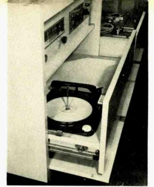
Fig. 6. No Tin Pan Alley is this vista of audio instrumentation, but rather a Rue de la Hi-Fi. Space alongside automatic record player is provided for addition of heavy-duty turntable in future. Control panel is recessed for knobs to clear doors when closed. Note spring catch in near edge of door.
