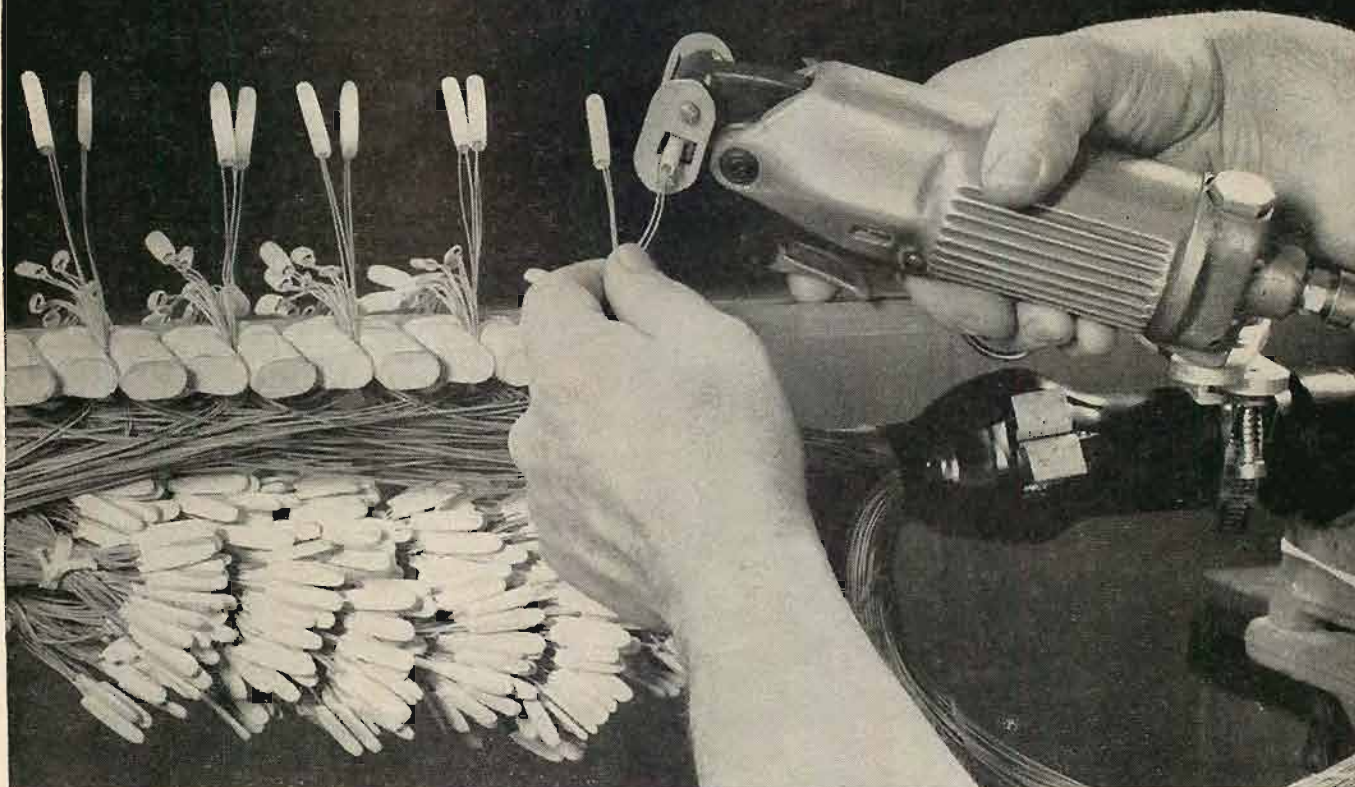
Telephone craftsman uses special pneumatic tool to flatten connector onto insulated wires. Metal tangs pierce insulation and produce a splice that is equivalent to a soldered joint.
