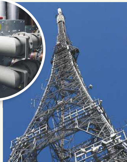
ABOVE: Equipment inside the BBC transmitter at Crystal Palace relies on waveguides (inset), which look more like plumbing than wiring
